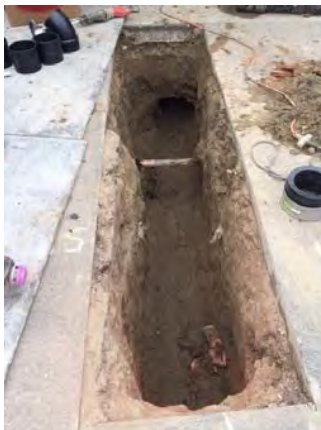
Trench with sewer Line removed
