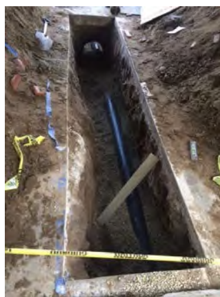
New sewer line installed.
