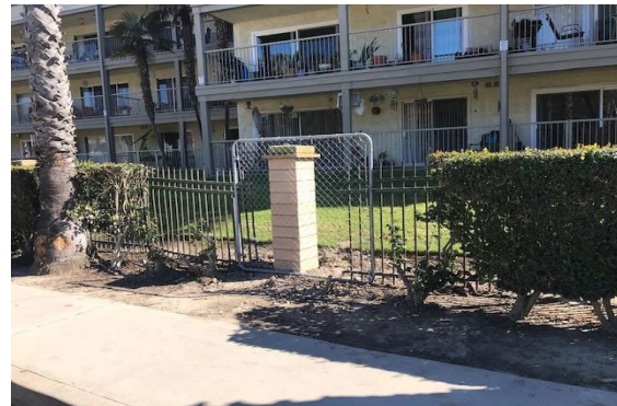
Current repair status
