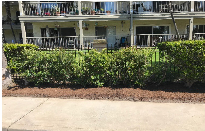
Replacement of fence, post and hedges
