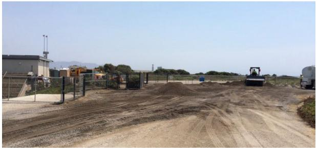
The County of Ventura is replacing the base material adjacent to their pump station due to structural issues with the base. They are now replacing the soil base with dirt and gravel to provide more support for all the heavy vehicles that visit the site.
