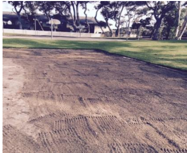
After work was completed!
