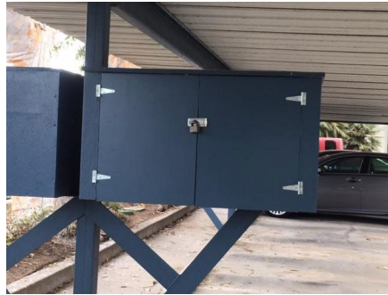
Replacement of carport storage boxes
