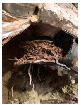
One, of the three unit stacks in Building 2 was experiencing blocked sewer drainage issues.
