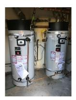
Two new water heaters have been installed in Building 7.
