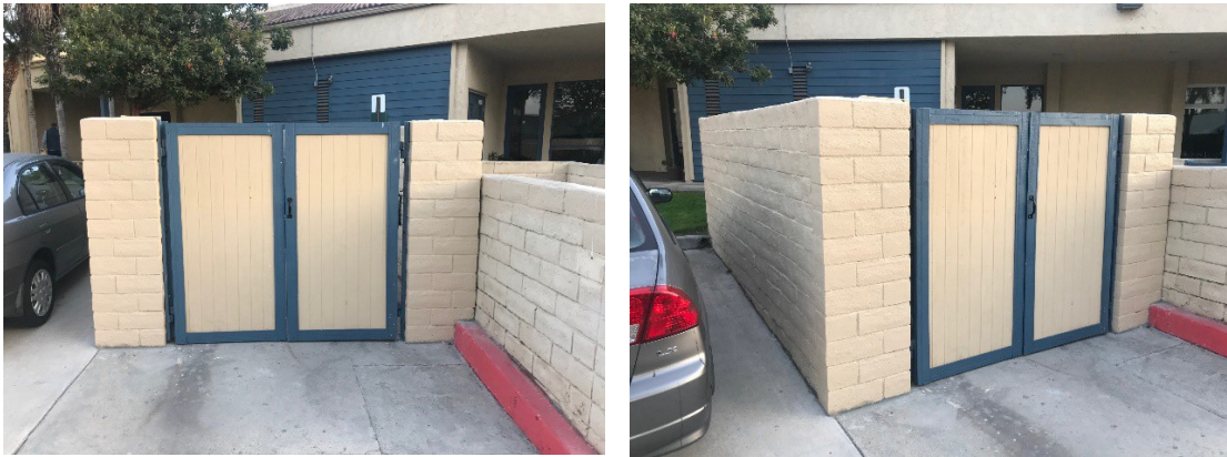
Trash enclosure with repairs completed.
