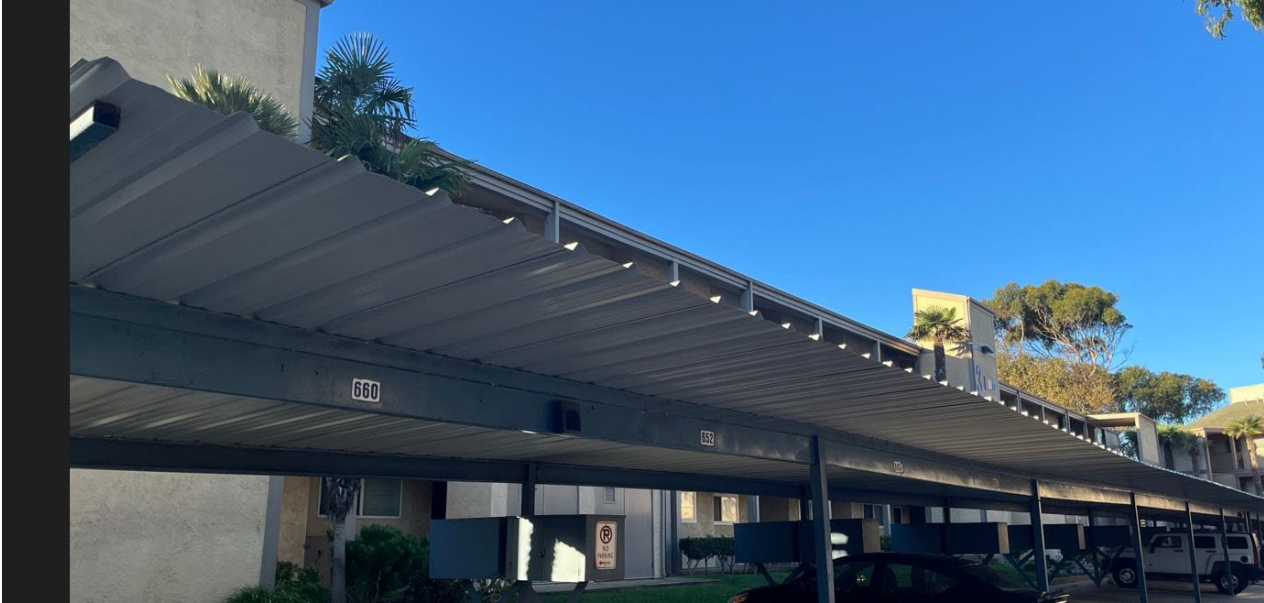
Replacement of Building 3 Carport Panels
