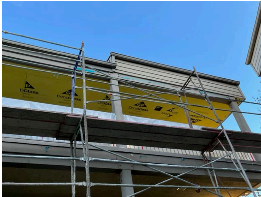
Ceiling Panels being Installed
