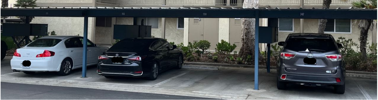
Replacement of Building 5 Carport Panels
