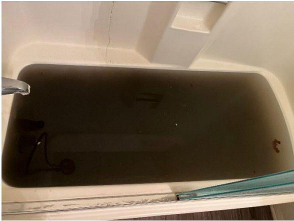
Water had been in tub for quite some time.
