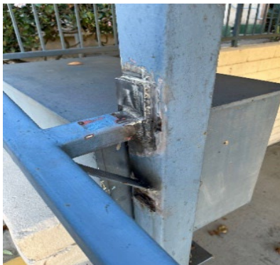
The handrail at Building 7 has been fixed.
