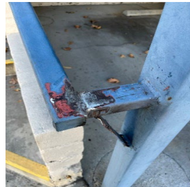
The handrail at Building 7 has been fixed.
