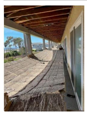
On **March 13, 2022**, the third-floor ceiling of building 3 collapsed. The replacement of this ceiling has been completed and very soon the remaining condo building ceilings will be reinforced.
