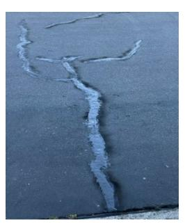
The recent heavy rains caused the street cracks to become larger. These cracks are now being treated with asphalt crack filler to prevent further damage to the street surface.
