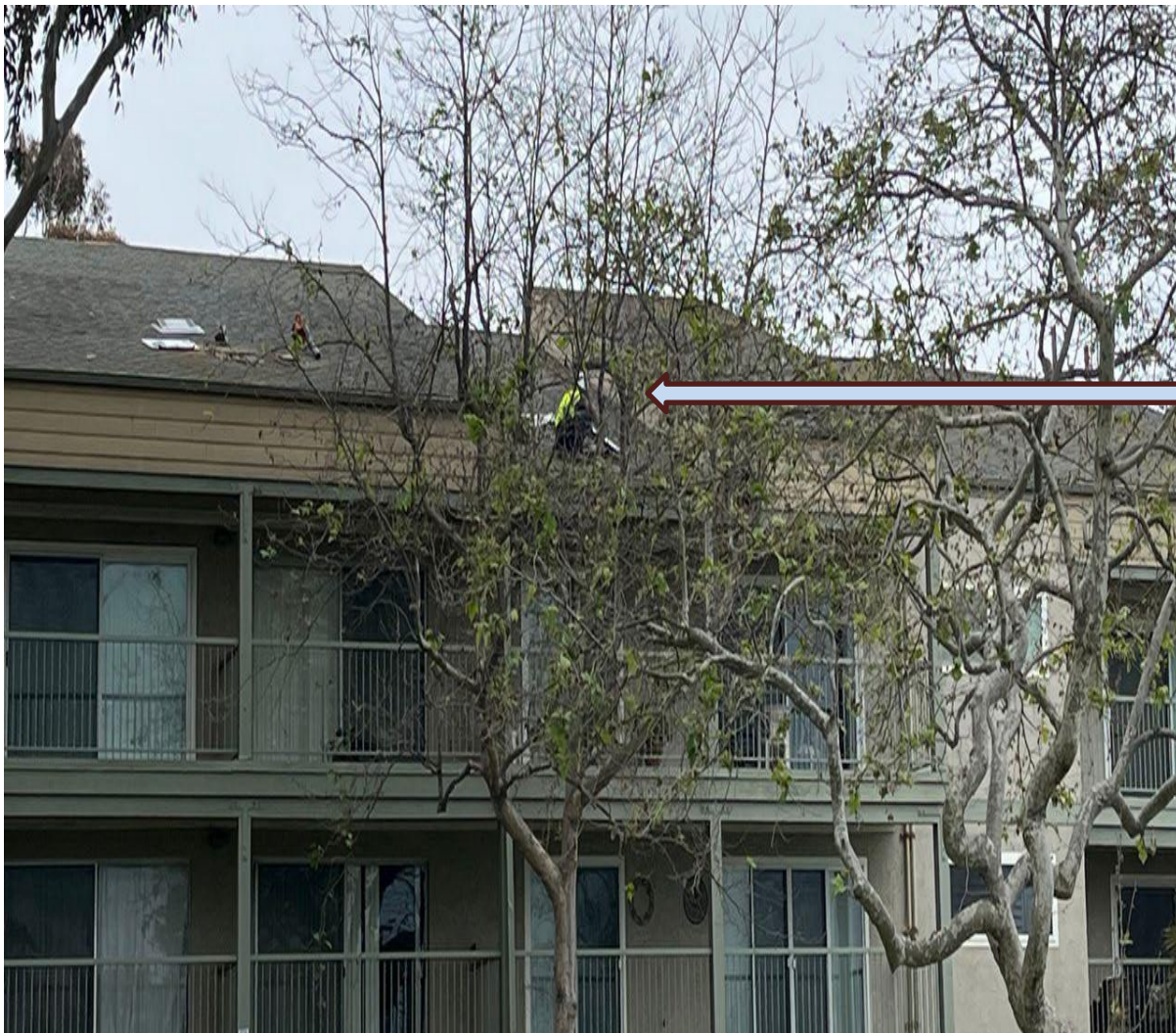
Vents being installed
