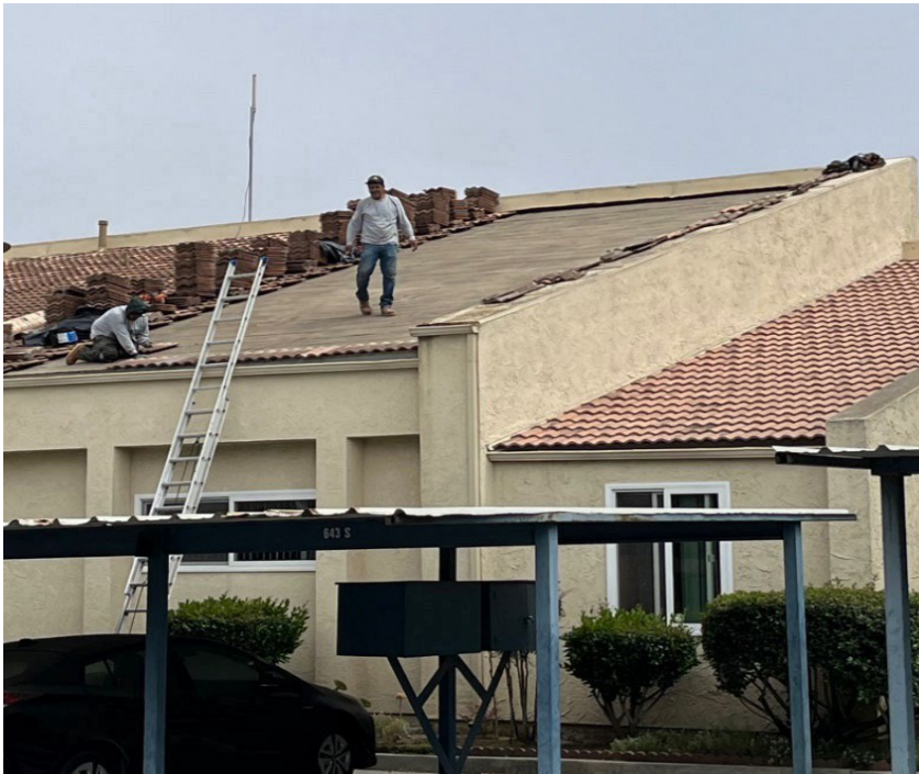
Clubhouse roof repair due to leaks caused by heavy rain.
