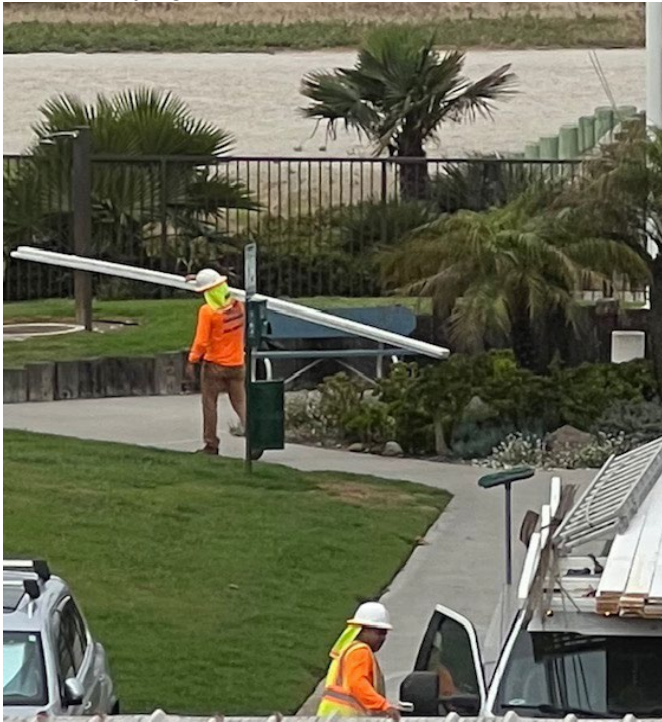
Carrying reinforcement wooden members
