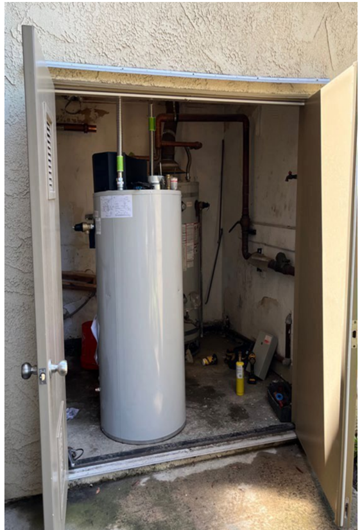
Building 5 water heater replacement
