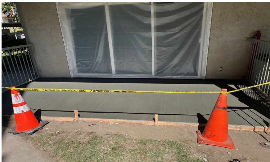
Slab being replaced due to structural issues.
