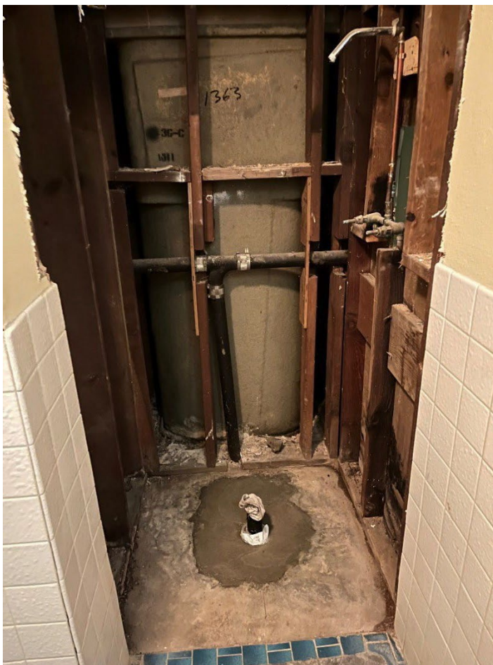
Women's bathroom in Clubhouse
