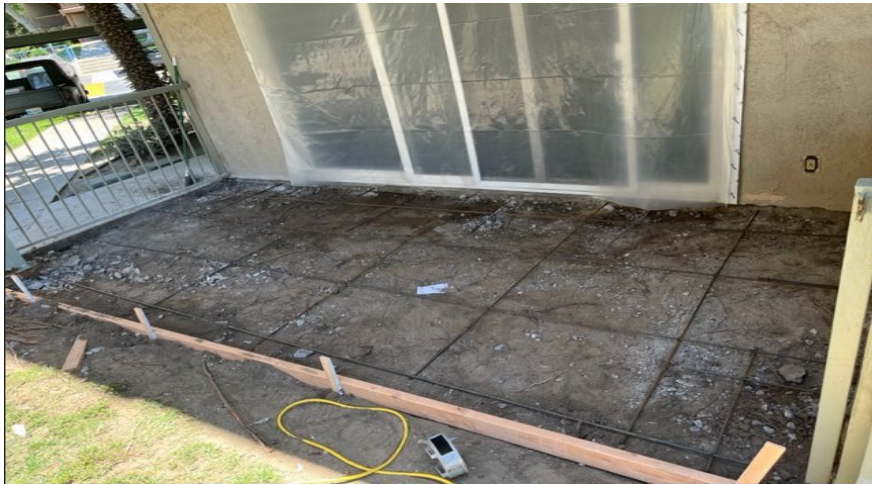
Slab being replaced due to structural issues.
