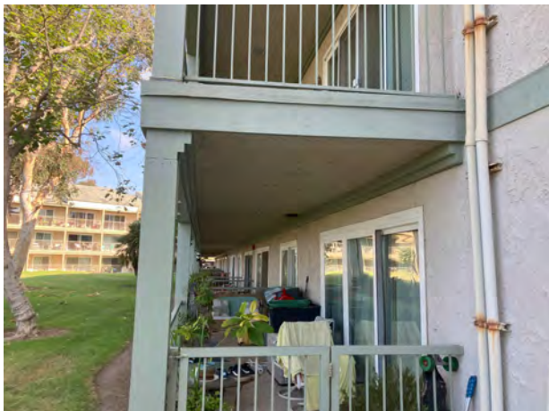
NEW LEDGER @ 1ST FLOOR SOFFIT - 09/25/23
