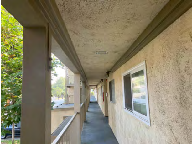
NEW LEDGER @ 2ND FLOOR SOFFIT - 09/25/23
