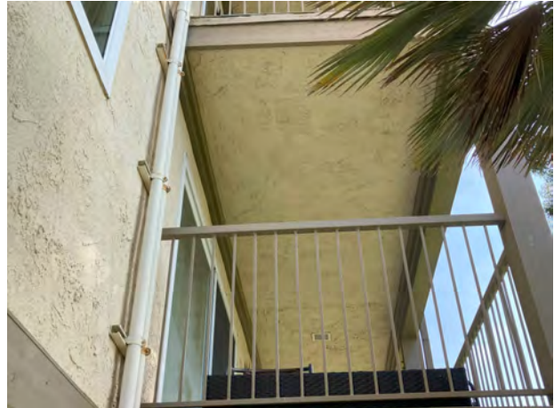
NEW LEDGER @ 2ND FLOOR SOFFIT - 09/25/23
