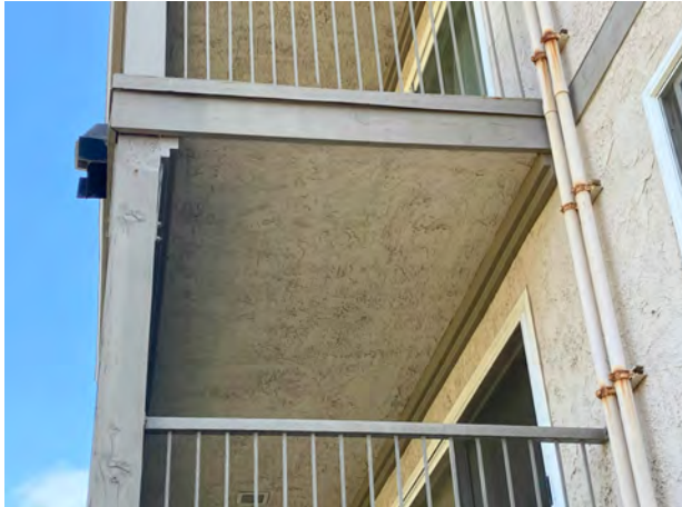
NEW LEDGER @ 2ND FLOOR SOFFIT - 09/25/23
