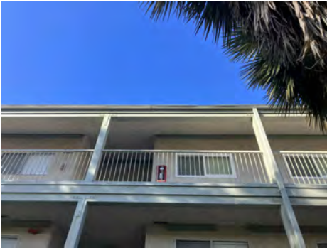
B. UNIT 824 - 3RD FLOOR 16' BEAM REPLACEMENT - 01-03-24
