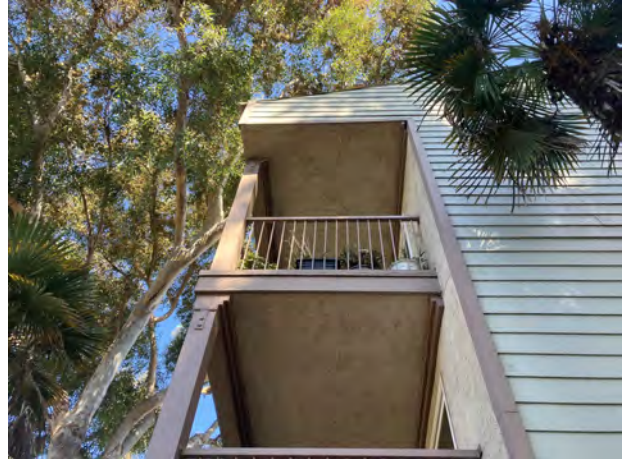
NEW LEDGER @ 3RD FLOOR SOFFIT - 10/23/23
