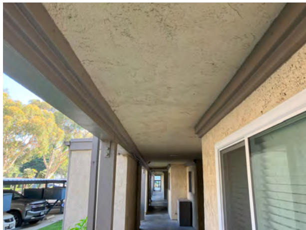
NEW LEDGER @ 1ST FLOOR SOFFIT - 09/25/23
