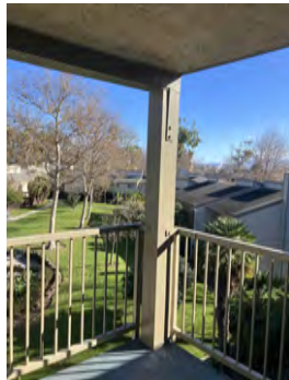
10. UNIT 669 - 3RD FLOOR ELEVATOR 8' POST REPLACEMENT - 01-03-24
