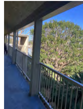
13. UNIT 663 - 3RD FLOOR 8' POST REPLACEMENT - 01-03-24
