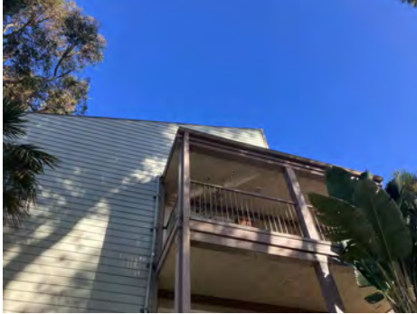
B. UNIT 664 - 3RD FLOOR 10' BEAM REPLACEMENT - 01-03-24
