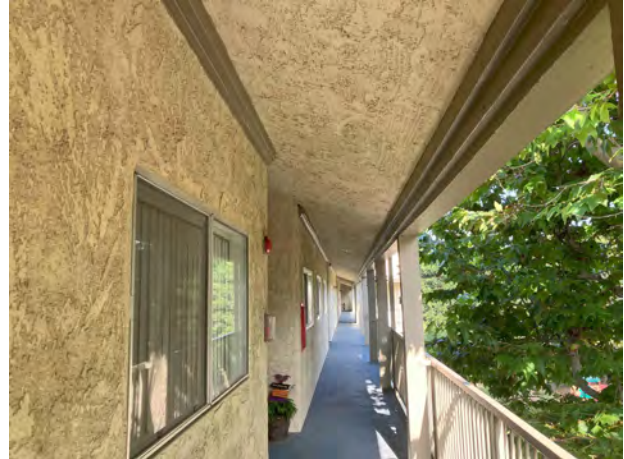
NEW LEDGER @ 3RD FLOOR SOFFIT - 09/25/23
