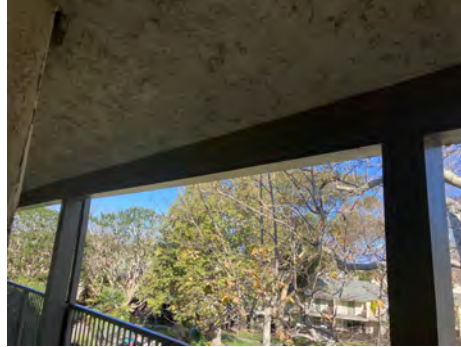
D. UNIT 687 - 3RD FLOOR 14' BEAM REPLACEMENT - 01-03-24
