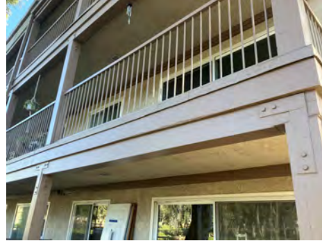
D. UNIT 660 - 1ST FLOOR 14' BEAM REPLACEMENT - 01-03-24
