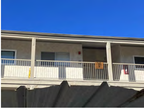
B. UNIT 661 - 3RD FLOOR 14' BEAM REPLACEMENT - 01-03-24
