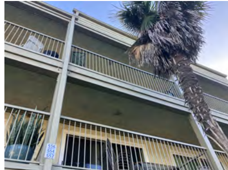
J. UNIT 554 - 2ND FLOOR 14' BEAM REPLACEMENT - 01-03-24
