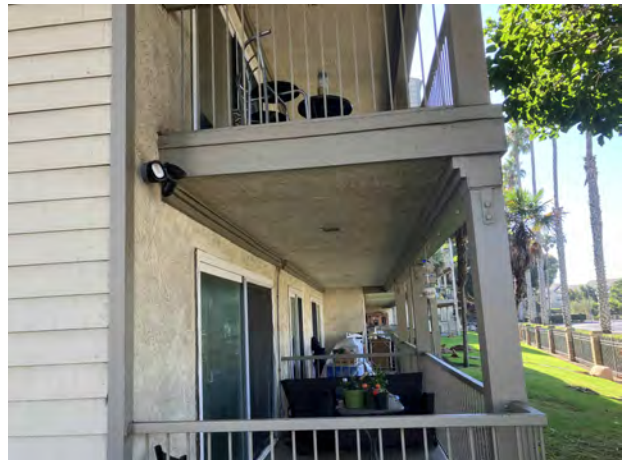
NEW LEDGER @ 1ST FLOOR SOFFIT - 10/23/23
