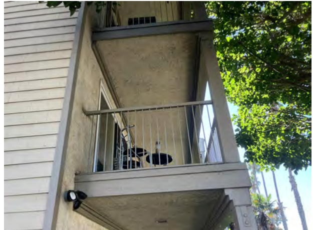
NEW LEDGER @ 2ND FLOOR SOFFIT - 10/23/23
