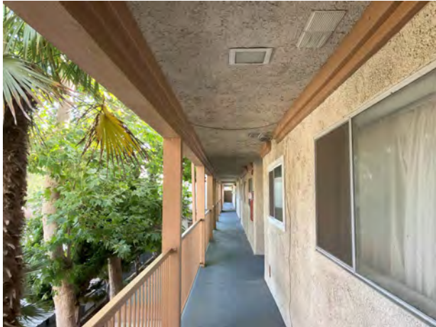
NEW LEDGER @ 2ND FLOOR SOFFIT - 09/25/23
