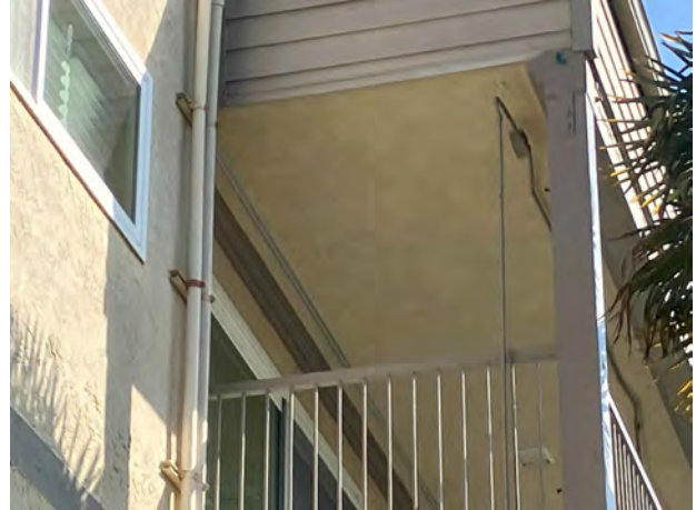
NEW LEDGER @ 3RD FLOOR SOFFIT - 09/25/23
