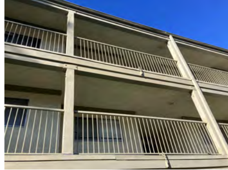
H. UNIT 524 - 2ND FLOOR 14' BEAM REPLACEMENT - 01-03-24
