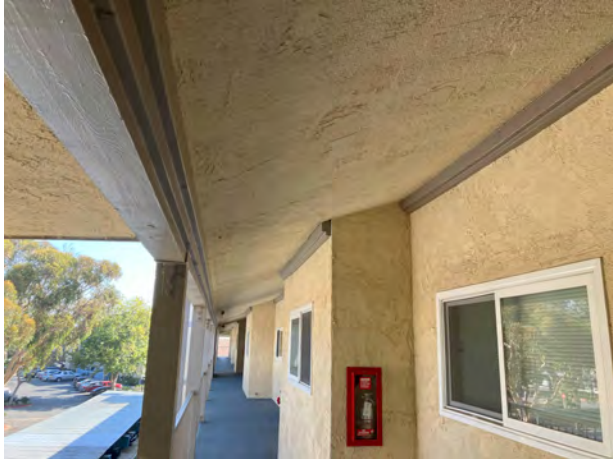
NEW LEDGER @ 3RD FLOOR SOFFIT - 09/25/23
