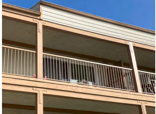
NEW LEDGER @ 3RD FLOOR SOFFIT - 09/25/23
