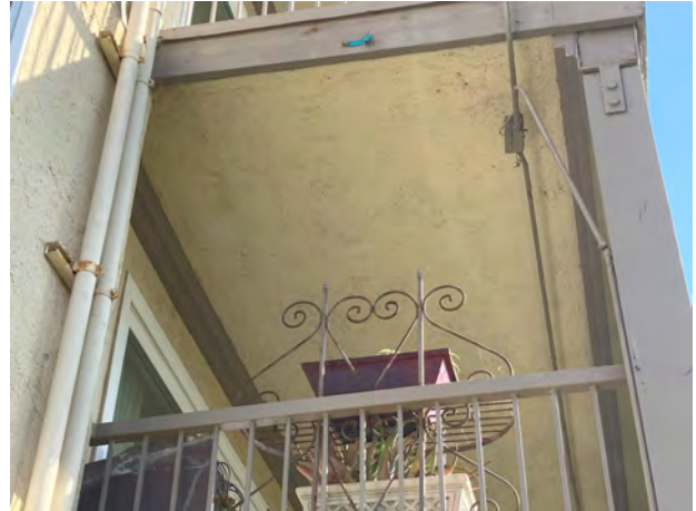
NEW LEDGER @ 2ND FLOOR SOFFIT - 09/25/23
