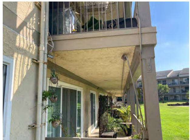
NEW LEDGER @ 1ST FLOOR SOFFIT - 09/25/23
