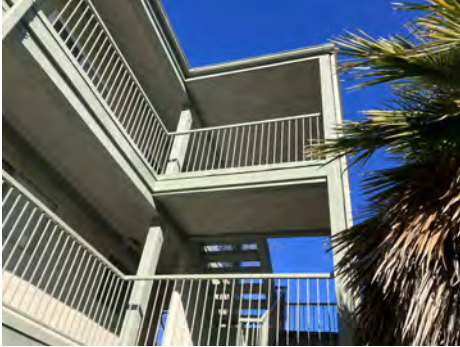
A. UNIT 864 - 2ND FLOOR 10' BEAM REPLACEMENT & STUCCO - 01-03-24
