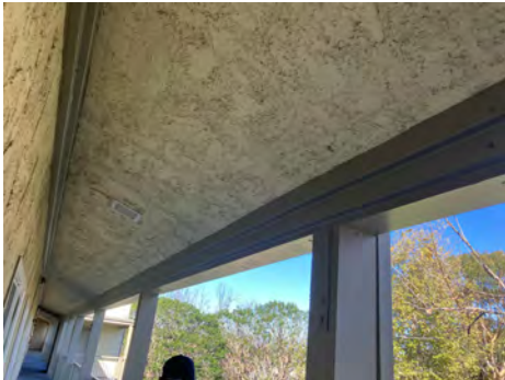
C. UNIT 687 - 3RD FLOOR 12' BEAM REPLACEMENT - 01-03-24
