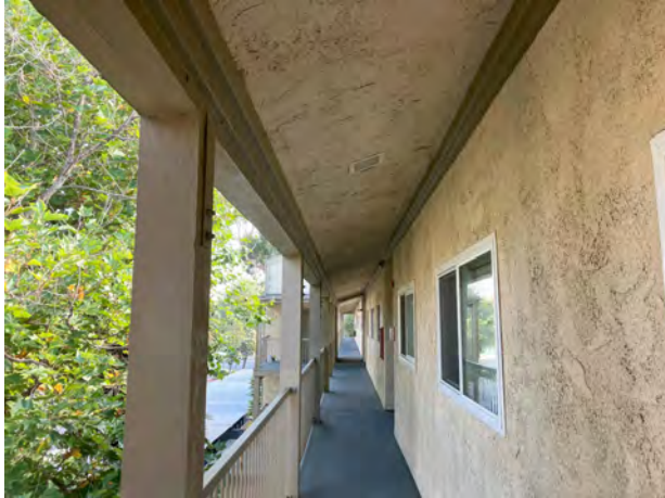
NEW LEDGER @ 3RD FLOOR SOFFIT - 09/25/23
