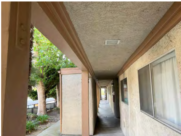
NEW LEDGER @ 1ST FLOOR SOFFIT - 09/25/23
