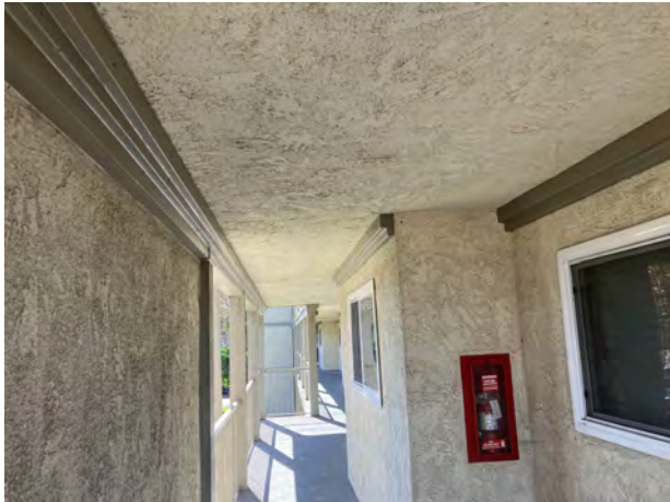
NEW LEDGER @ 2ND FLOOR SOFFIT - 10/23/23
