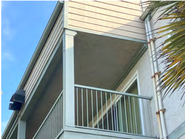
NEW LEDGER @ 3RD FLOOR SOFFIT - 09/25/23
