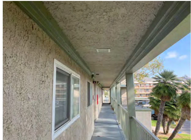
NEW LEDGER @ 2ND FLOOR SOFFIT - 09/25/23
