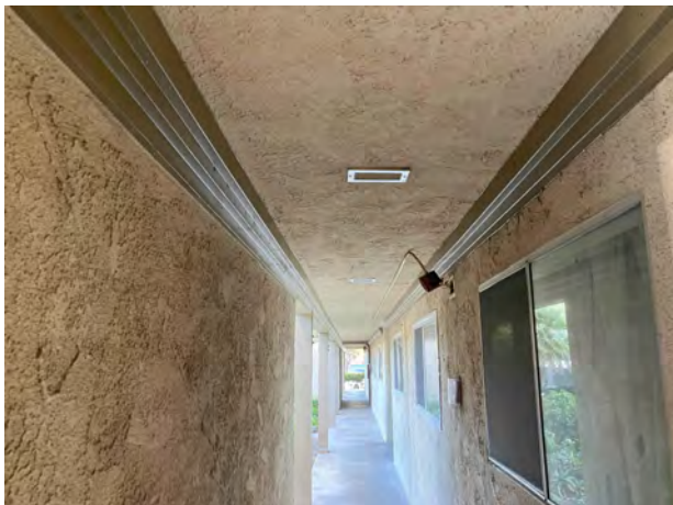
NEW LEDGER @ 1ST FLOOR SOFFIT - 09/25/23
