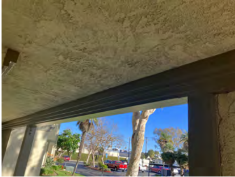
D. UNIT 566 - 1ST FLOOR STAIRWELL 16' BEAM REPLACEMENT - 01-03-24
