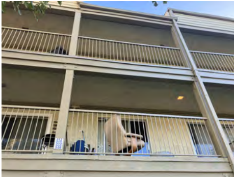
E. UNIT 510 - 2ND FLOOR 12' BEAM REPLACEMENT - 01-03-24
