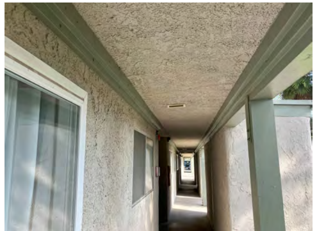
NEW LEDGER @ 1ST FLOOR SOFFIT - 09/25/23
