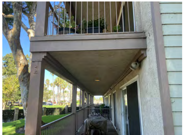
NEW LEDGER @ 1ST FLOOR SOFFIT - 10/23/23
