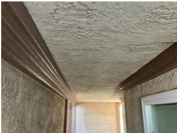
NEW LEDGER @ 1ST FLOOR SOFFIT - 10/23/23
