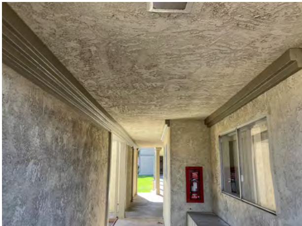
NEW LEDGER @ 1ST FLOOR SOFFIT - 10/23/23
