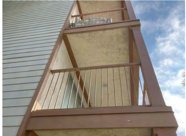
NEW LEDGER @ 2ND FLOOR SOFFIT - 09/25/23
