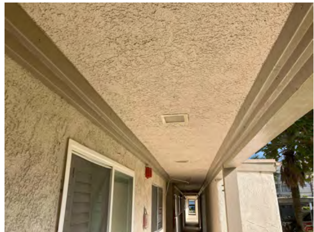
NEW LEDGER @ 1ST FLOOR SOFFIT - 09/25/23
