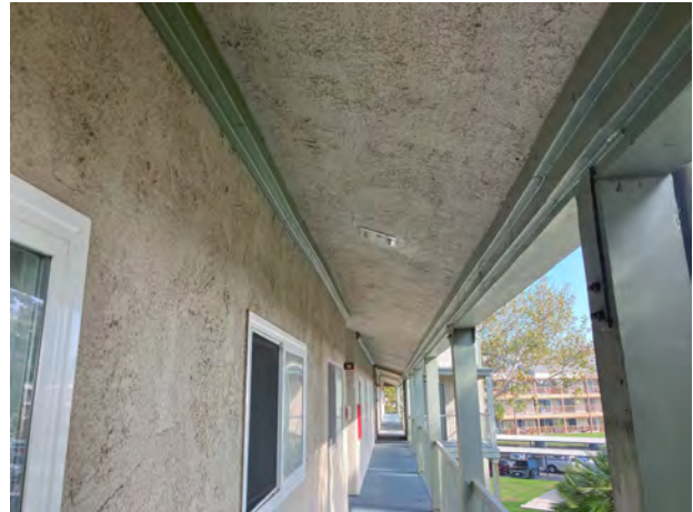
NEW LEDGER @ 3RD FLOOR SOFFIT - 09/25/23
