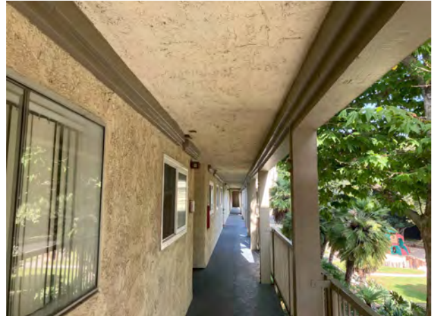
NEW LEDGER @ 2ND FLOOR SOFFIT - 09/25/23
