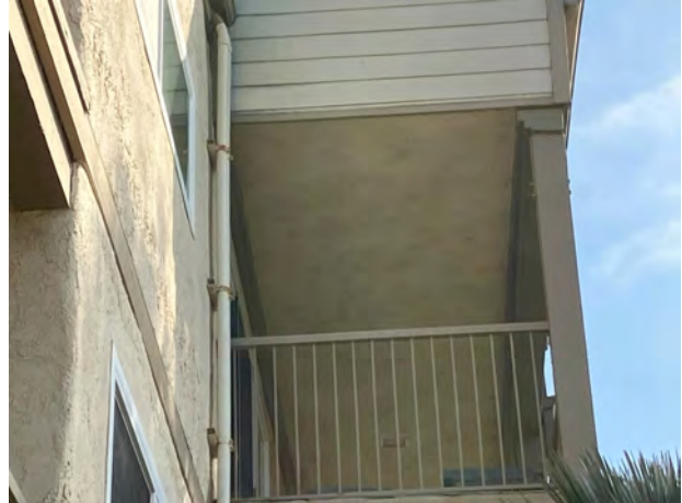
NEW LEDGER @ 3RD FLOOR SOFFIT - 09/25/23
