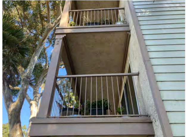
NEW LEDGER @ 2ND FLOOR SOFFIT - 10/23/23
