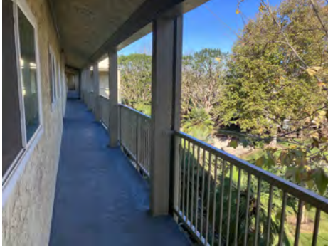
9. UNIT 687 - 3RD FLOOR 8' POST REPLACEMENT - 01-03-24
