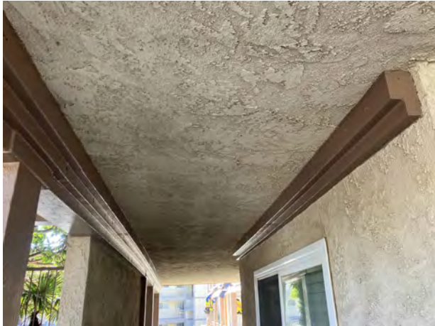
NEW LEDGER @ 2ND FLOOR SOFFIT - 10/23/23
