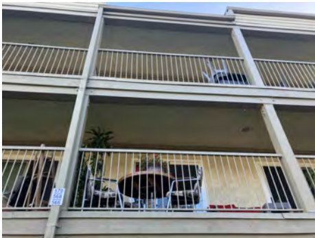
F. UNIT 568 - 2ND FLOOR 12' BEAM REPLACEMENT - 01-03-24
