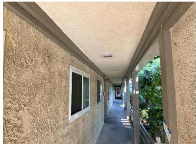
NEW LEDGER @ 1ST FLOOR SOFFIT - 09/25/23
