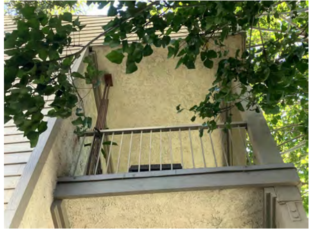
NEW LEDGER @ 3RD FLOOR SOFFIT - 10/23/23
