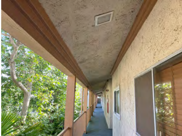
NEW LEDGER @ 3RD FLOOR SOFFIT - 09/25/23
