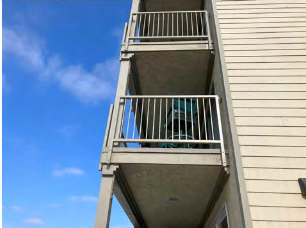
NEW LEDGER @ 2ND FLOOR SOFFIT - 09/25/23
