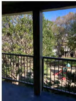
11. UNIT 651 - 3RD FLOOR 8' POST REPLACEMENT - 01-03-24
