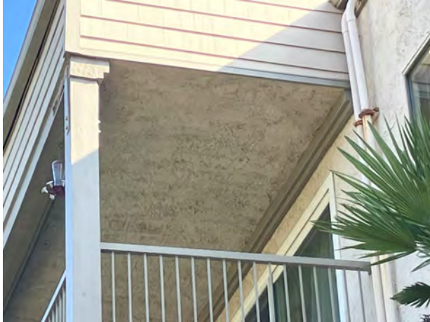
NEW LEDGER @ 3RD FLOOR SOFFIT - 09/25/23
