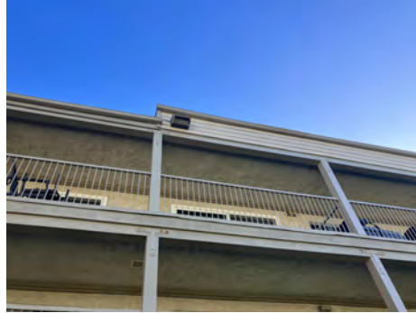
C. UNIT 667 - 3RD FLOOR 12' BEAM & 5. UNIT 667 3RD FLOOR 8' POST REPLACEMENT - 01-03-24
