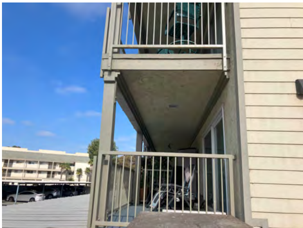
NEW LEDGER @ 1ST FLOOR SOFFIT - 09/25/23
