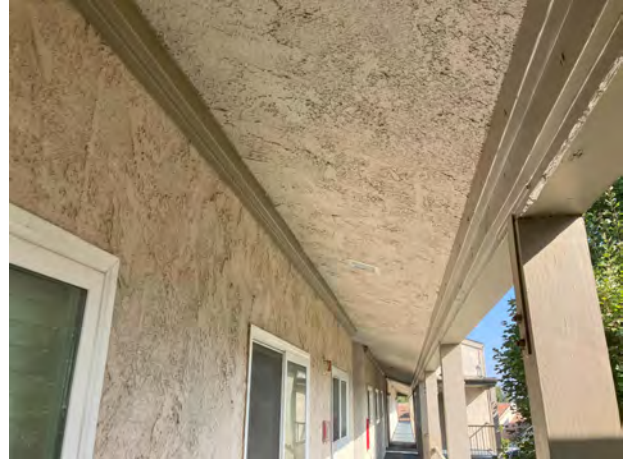
NEW LEDGER @ 3RD FLOOR SOFFIT - 09/25/23
