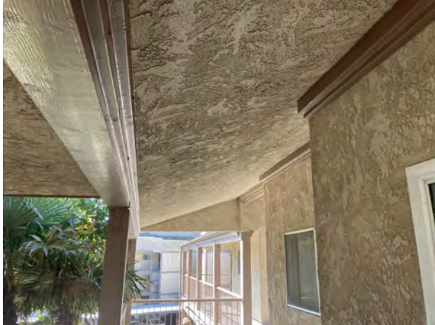
NEW LEDGER @ 3RD FLOOR SOFFIT - 10/23/23
