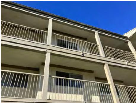
G. UNIT 526 - 2ND FLOOR 12' BEAM REPLACEMENT - 01-03-24
