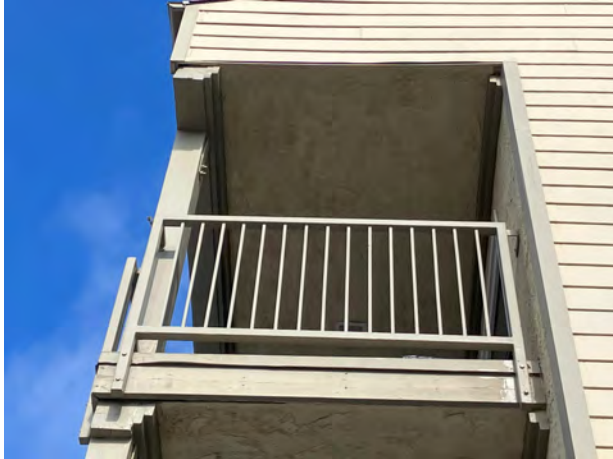
NEW LEDGER @ 3RD FLOOR SOFFIT - 09/25/23
