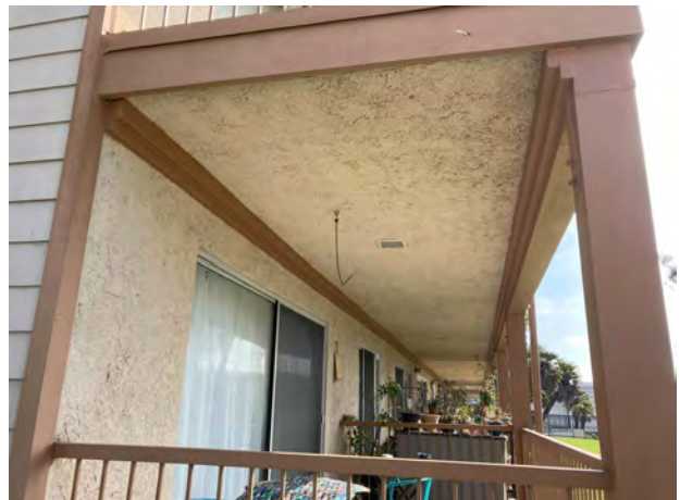
NEW LEDGER @ 1ST FLOOR SOFFIT - 09/25/23
