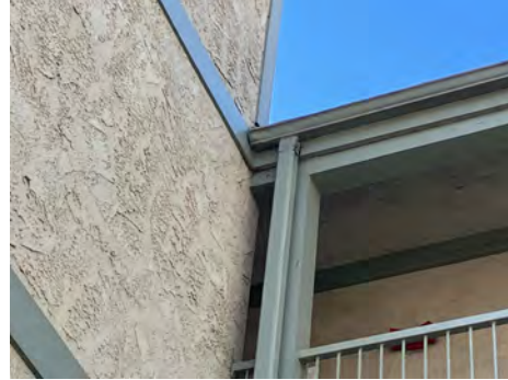
C. UNIT 836 - 3RD FLOOR 1' BEAM REPLACEMENT - 01-03-24
