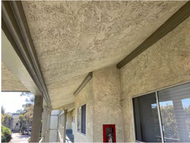
NEW LEDGER @ 3RD FLOOR SOFFIT - 10/23/23
