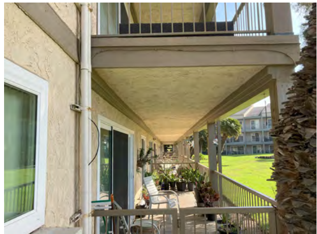
NEW LEDGER @ 1ST FLOOR SOFFIT - 09/25/23
