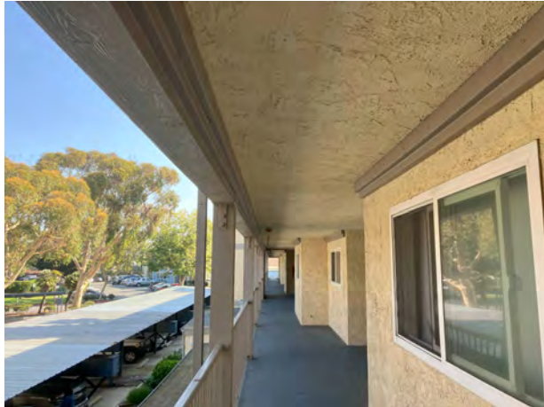
NEW LEDGER @ 2ND FLOOR SOFFIT - 09/25/23
