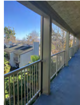
12. UNIT 669 - 3RD FLOOR 8' POST REPLACEMENT - 01-03-24
