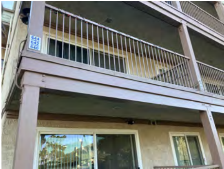
C. UNIT 640 - 1ST FLOOR 14' BEAM REPLACEMENT - 01-03-24
