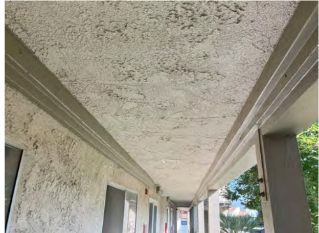
NEW LEDGER @ 2ND FLOOR SOFFIT - 09/25/23
