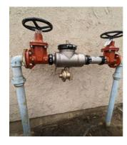
A new irrigation backflow valve was installed by building 7. This device will protect the water quality in the system.
