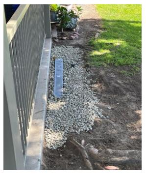
The rainwater was not able to drain properly because the adjacent tree roots acted as a dam.
