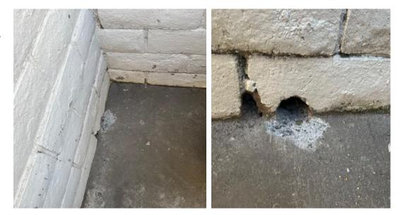
A drain hole was made in the refuse wall site, a pipe was installed on the opposite side, and the rainwater is now able to drain directly into the street.
