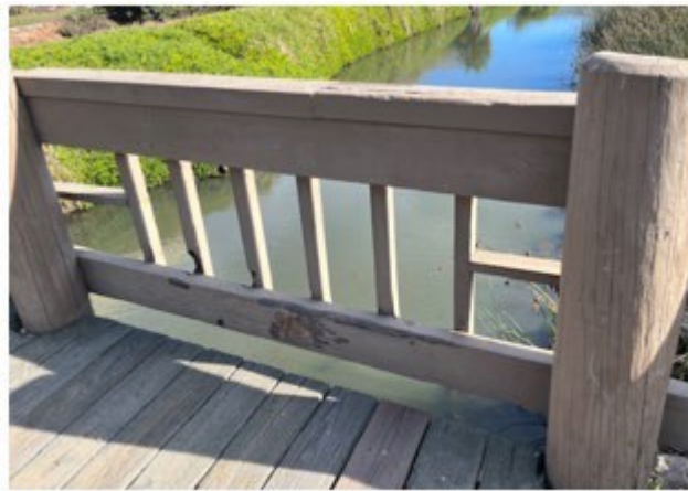
Existing Bridge Railing
