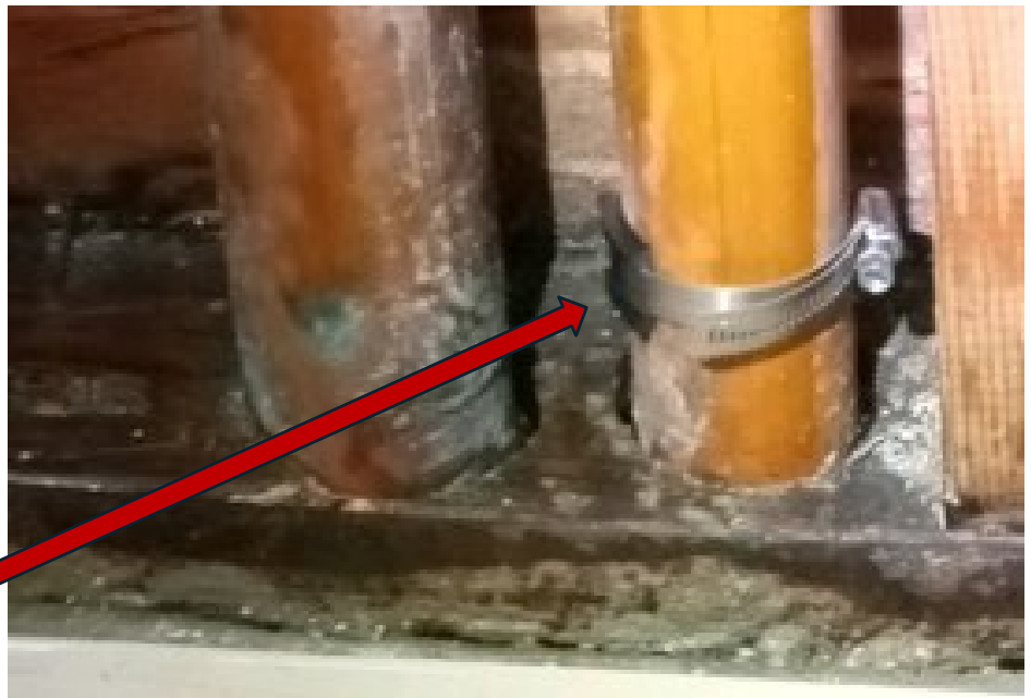
Plugged pinhole in pipe is where the bracket is located.
