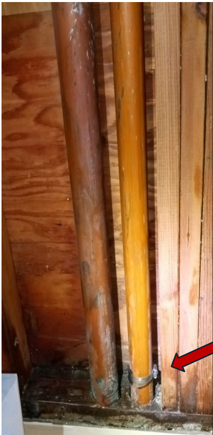
Plugged pinhole in pipe is where the bracket is located.
