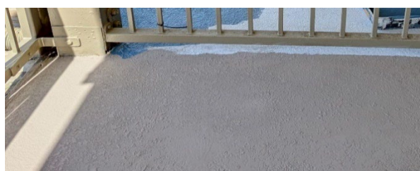
Repaired balcony prior blue paint overcoat
