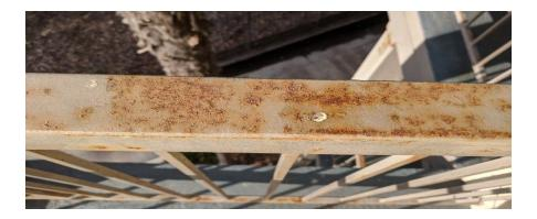
Untreated rust areas will eat through the paint and damage the integrity of the railings.
