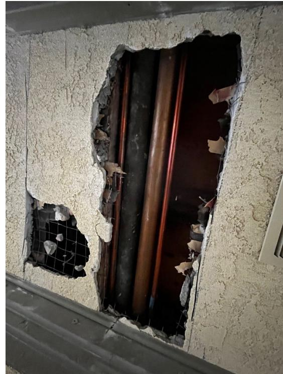
Over twelve years ago, the sewer lines in the structures were replaced due to breakage, leakage, and bonding. At the same time, the inside of the water lines were coated with epoxy to minimize pinhole leaks. Through time and use, some of the epoxy has become loose and has started blocking the flow of water.
